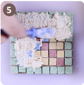
Use a glue spreader to press grout into the interstices.
